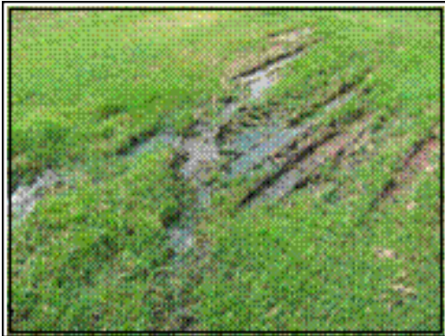
The leachfield from a failed septic system, from aero-stream.com
